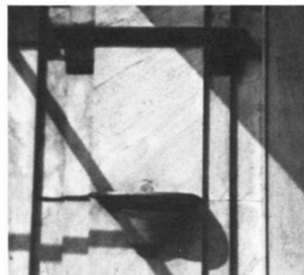
26 Terragni, Hotel Metropole-Suisse, detail of pilaster capitals
